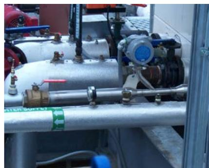
A 454FTB WGF unit was installed to measure output from the acid fermentation tank.
