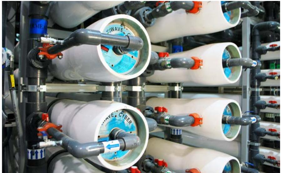
*Pre-treatment removes contaminants, which helps the RO membranes resist fouling.*
