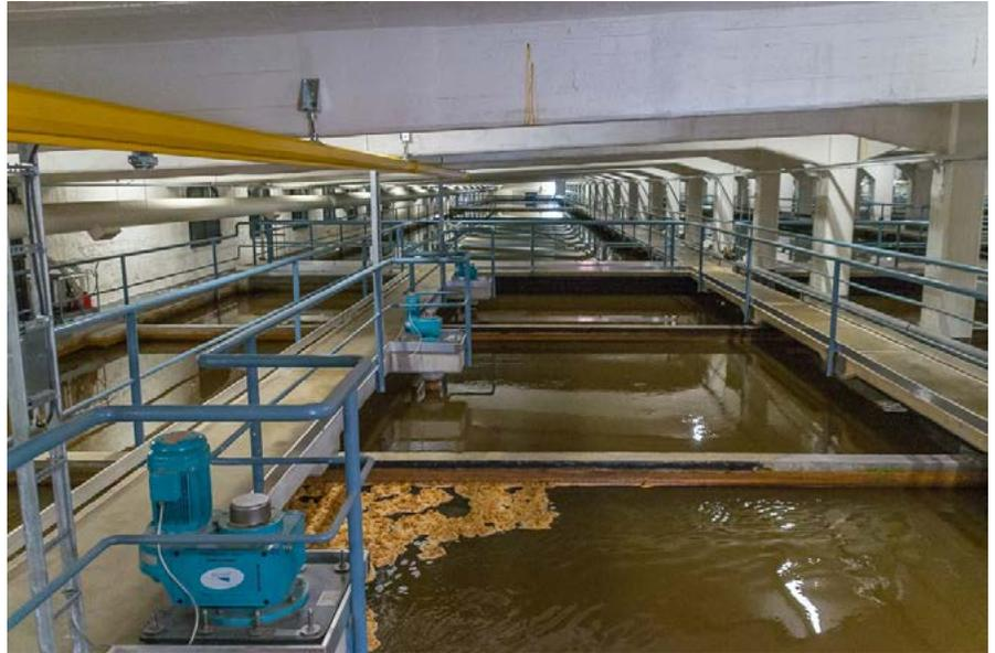
INVENT Hyperclass<sup>®</sup> mixers in the flocculation tank
