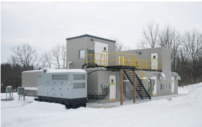
The Newterra fully-clad system in the small Township of Southwold, came complete with odor & noise attenuation, due to its proximity to the development and surrounding green space. The first system was designed with a capacity of 500 m 3 /day (132, 000 GPD), with the option of being expandable to 1,200 m 3 /day (317, 000 GPD).
