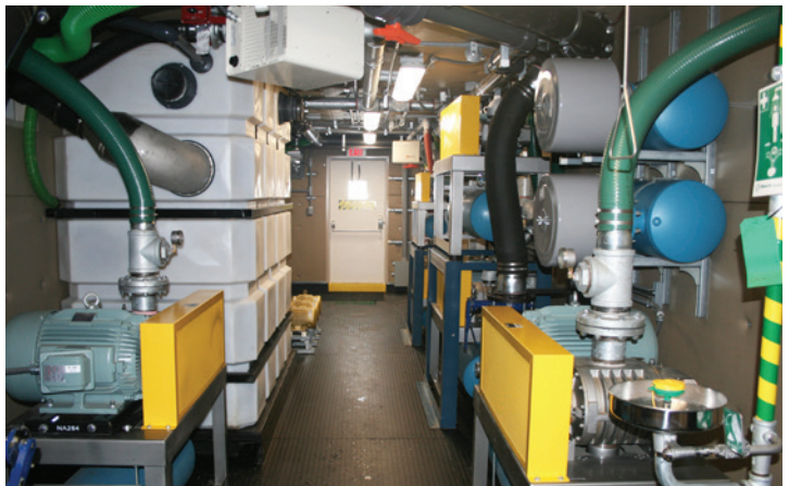
The Newterra fully-clad system in the small Township of Southwold, came complete with odor & noise attenuation, due to its proximity to the development and surrounding green space. The first system was designed with a capacity of 500 m 3 /day (132, 000 GPD), with the option of being expandable to 1,200 m 3 /day (317, 000 GPD).
