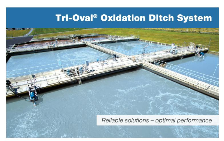
The Newterra Tri-Oval® Oxidation Ditch System, named for our Triton in an oxidation oval, is a subsurface complete mix, looped reactor system that is ideal for municipal and industrial wastewater treatment facilities. The energy efficient Triton TR Series process aerator/mixer, combined with an optimized control strategy, allows for operation at depths as low as 4ft (1.22m) and up to 33ft (10m).
