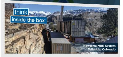
**Scalable:** Our modular systems can expand as capacity requirements change – and be redeployed at the end of a temporary project if necessary. Developers can defer infrastructure spending by phasing in sewage treatment capacity in parallel with the phases of a project.
