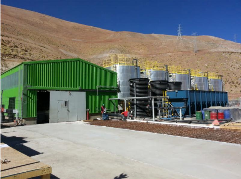
In late 2013 **newterra** was contracted to design, build and rapidly deploy a modular and pre-manufactured 10 liter per second metals precipitation and solids removal system for a copper mine in Chile.
