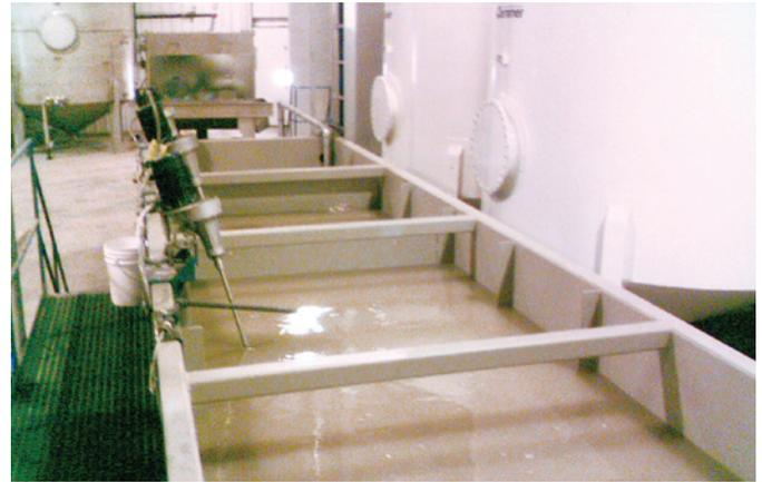
carbon contactor vessel. Filter Innovations virgin activated carbon made from the finest grades of bituminous coal, it is ideal for many liquid phase applications including the removal of organics from water streams and the purification of potable water.
