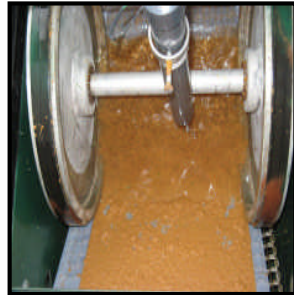
Dewatering of coagulated iron in the automatic particulate filter
