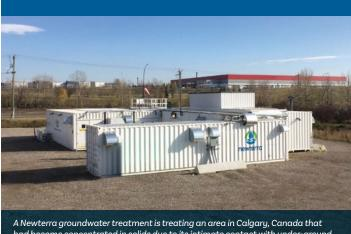
A Newterra groundwater treatment is treating an area in Calgary, Canada that had become concentrated in solids due to its intimate contact with under-ground minerals over time. The treated water is then discharged back into the environment
